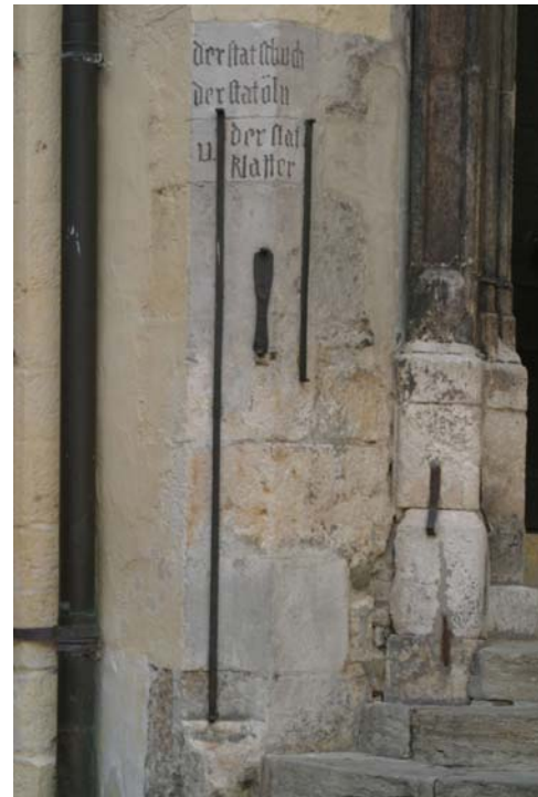
Figure 2. Above: Measurement standards embedded in the wall of the city hall in Assisi, Italy. The measurements are the foot, the cubit, and the yard. Right: Measurements in the wall of the city hall in Regensburg, Germany. The measurements are the foot, the yard, and the fathom.
